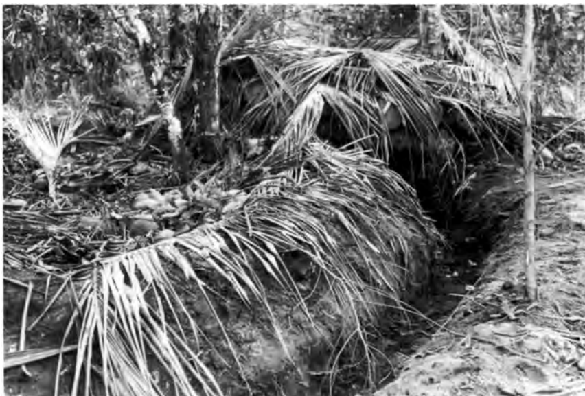
Coconut log bunker with fire trench entrance in the Buna Village area. (DA photograph)
